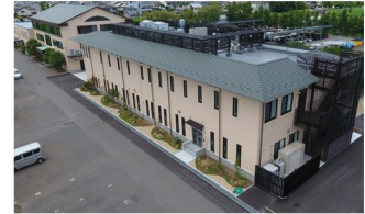
New Testing Building
